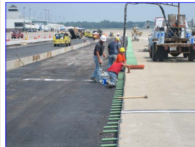
Crews working on Job 21.
