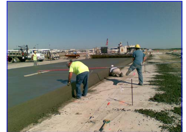
Crews working on Job 22.
